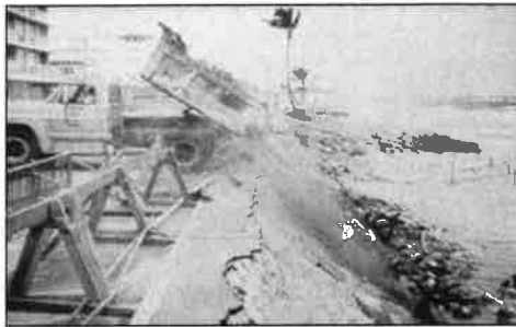
Figure 35. Emergency dumping of riprap to protect a coastal highway at Delray Beach threatened by erosion during storms (courtesy of Coastal Planning and Engineering Inc.).
