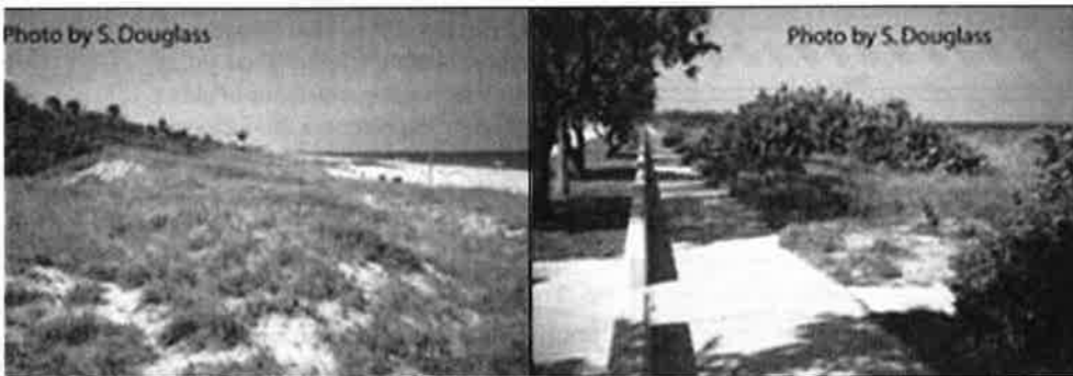
Figure 38 (below). Delray Beach revetment after beach nourishment (Federal Highway Administration 2012).
