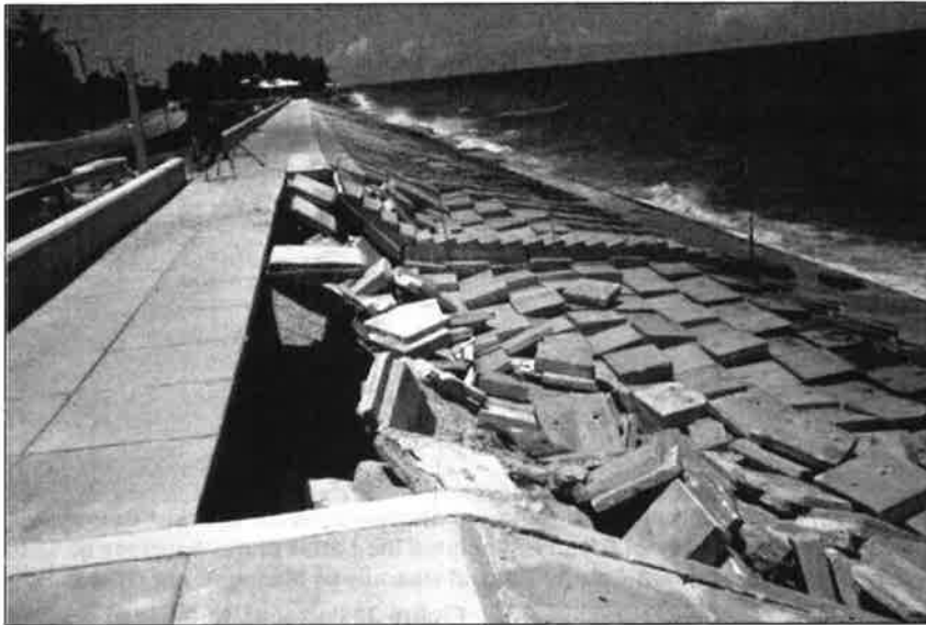
Figure 36. Damaged interlocking concrete revetment. Photograph from the early 1970s (courtesy of Robert G. Dean).
